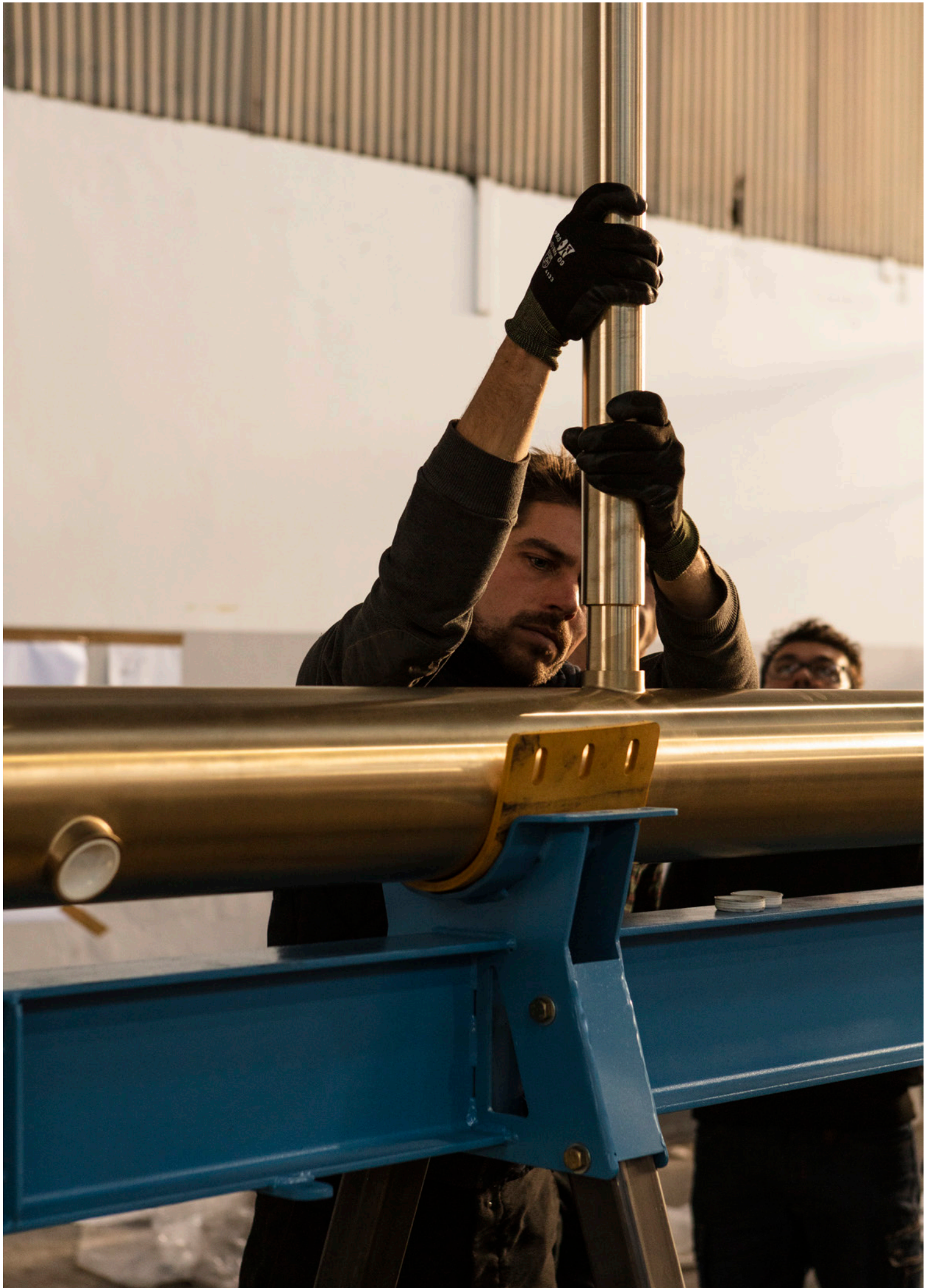
Assembly of the fountain masts
